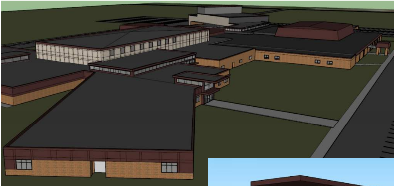
View of Building Addition from the Southwest
